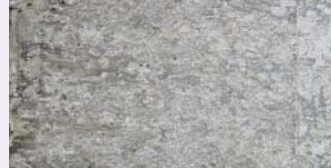
Untreated Panels corrode rapidly.
